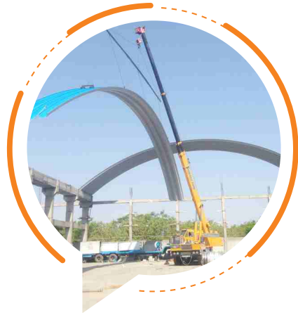
Crane Setup & Installation
